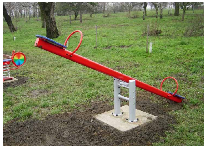
In addition to having unacceptable surfacing around it, this seesaw's exposed concrete footing and potential pinch point poses a hazard to children.
