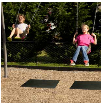
Wear Mats under swings can help keep loose-fill materials in place and protect unitary surfaces from wear.
