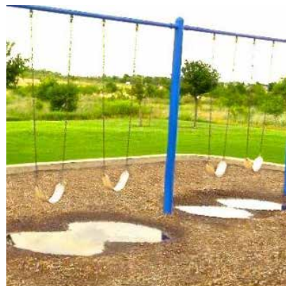
Loose-fill materials get kicked away and must be raked level.
