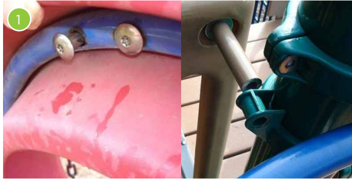
1 This bolt is loose and should be tightened or replaced.
