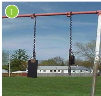
Swing chain should be unwrapped/inspected and broken swing seat should be replaced.
